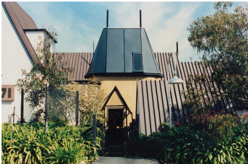
Figure 4: East-side View of the Hunsbury House, 1991
